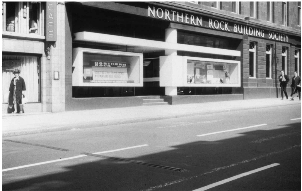
Figure 7. Northern Rock Building Society, Newcastle, 1964.
