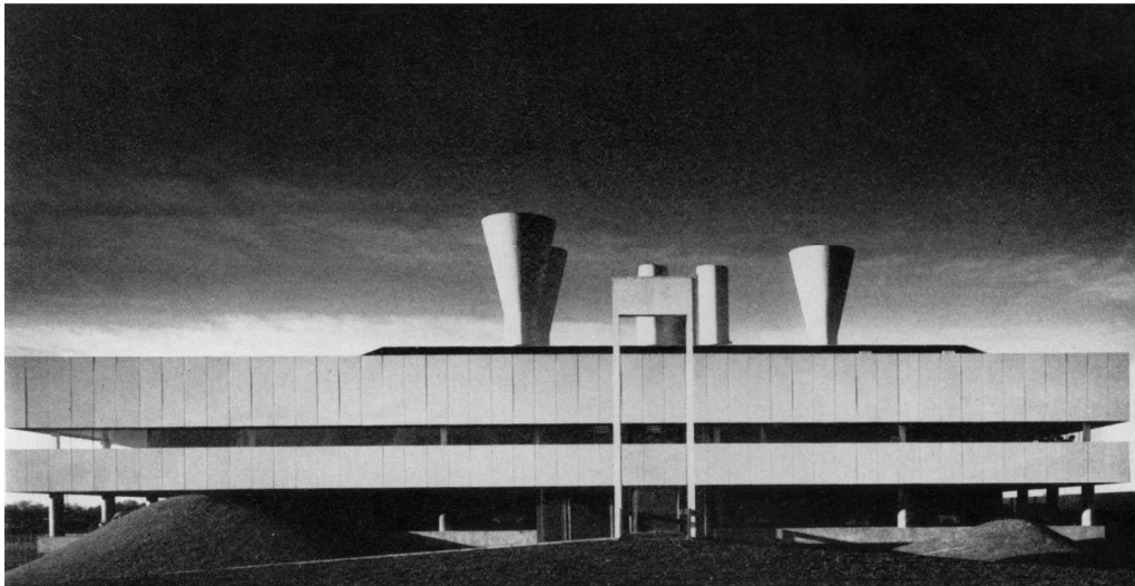
Figure 10. Gas Council Engineering Research Station, Killingworth, Northumberland, 1967.
