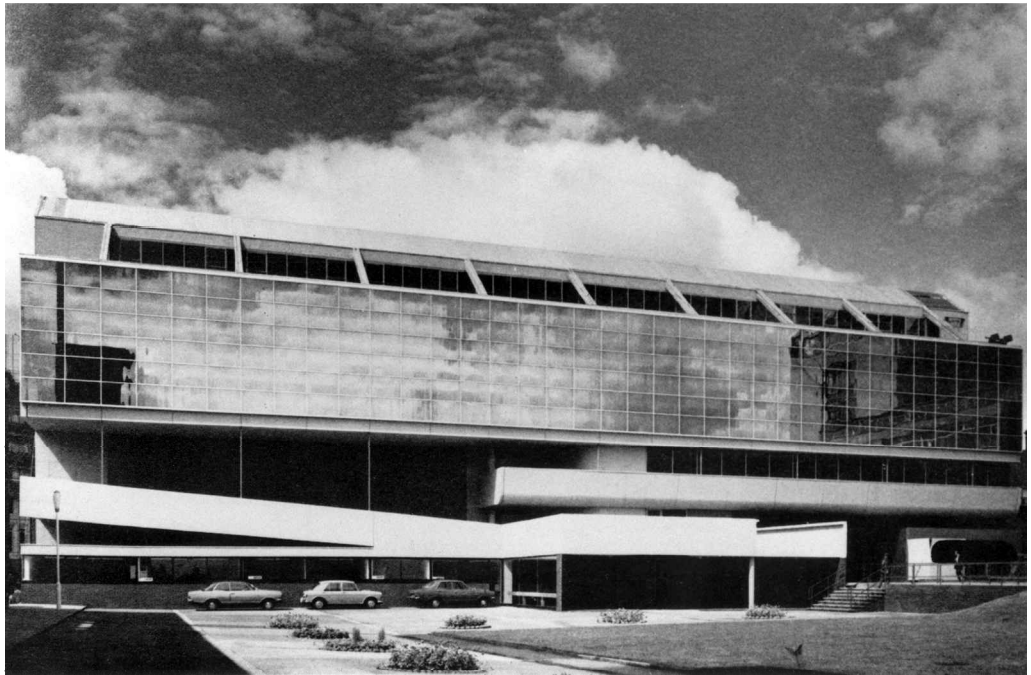
Figure 13. MEA building, Newcastle, 1974.
